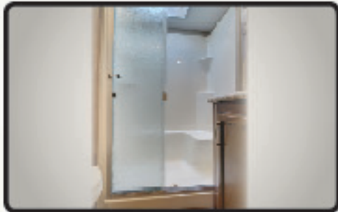
SEAMLESS 48"X30" FIBERGLASS SHOWER W/SEAT, NOT 2PC. PLASTIC
